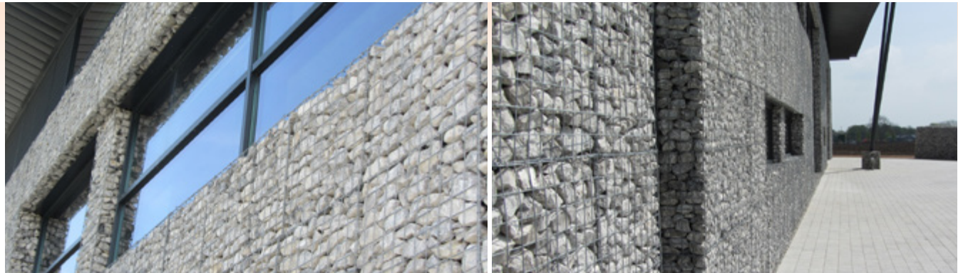
As these photos illustrate, the exterior and interior walls of the Nestlé Waters building show the success with which architectural features can be emphasised—using a combination of gabion mesh systems supplied by Enviromesh—and carefully specified aggregate/filling material
